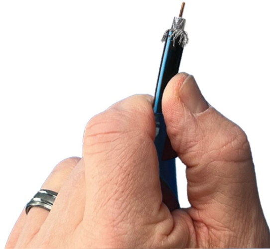
Figure 56: Folding the inner braid against the folded outer braid
