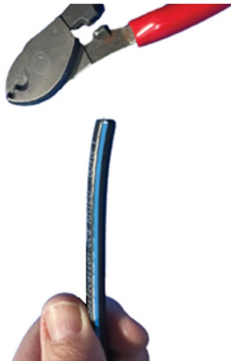
Figure 47: Cutting the IFL cable to length
