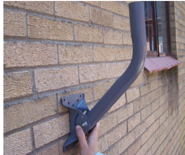
Figure 28: Pole assembly
