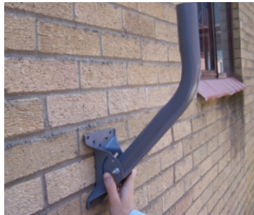
Figure 30: Pole assembly
