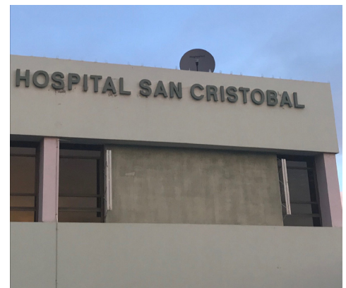
A Hughes VSAT solution installed on the roof of the Hospital San Cristobal made connectivity possible.
